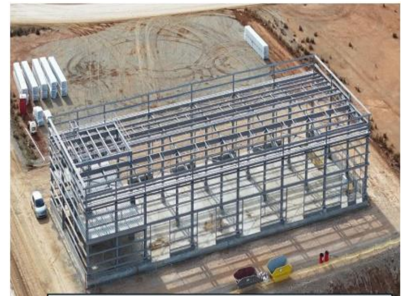
Maintenance Building Structural steel Works
