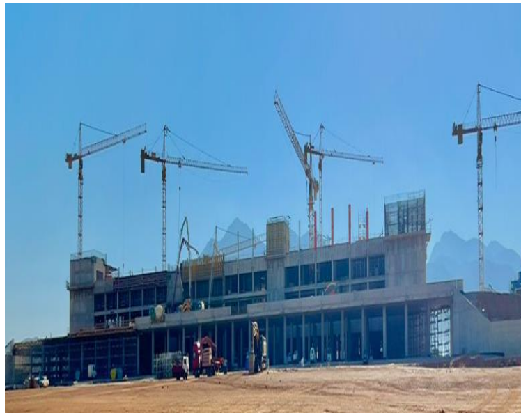
Terminal Building Structural Concreting works
