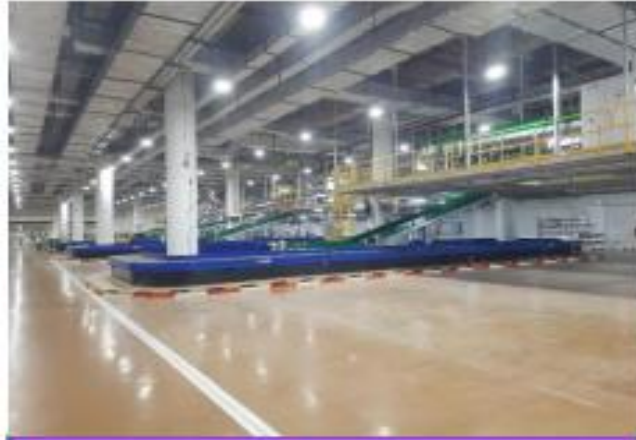
Baggage Handling Works
