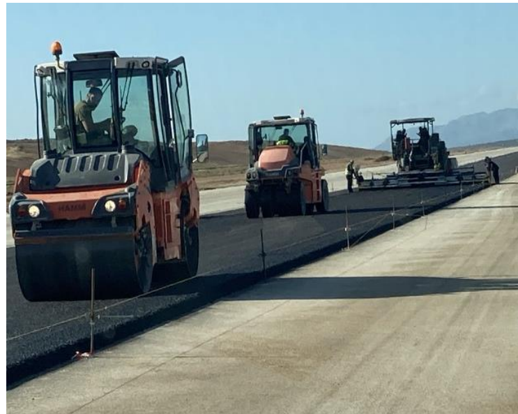
Taxiway Asphalt Paving
