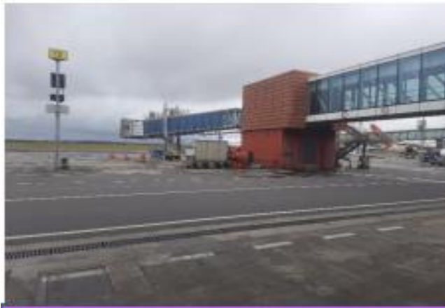
Passenger Boarding Bridge
