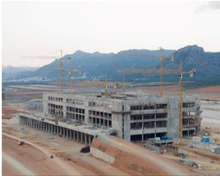
Terminal Building Structural Concreting works
