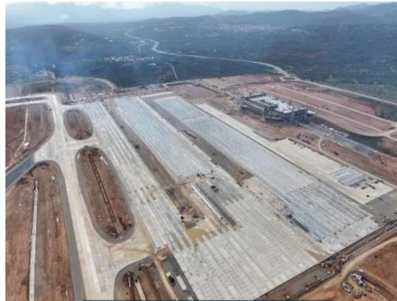
Apron Pavement and Ground Power Unit Works
