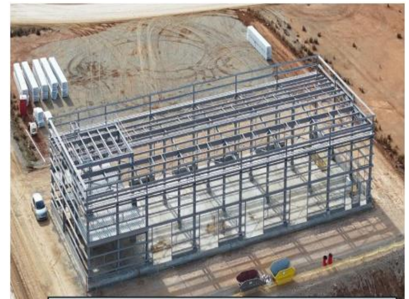
Maintenance Building Structural steel Works
